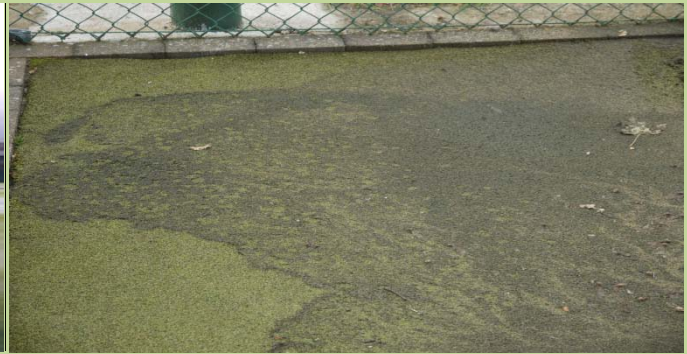
Algal Growth Can Be Evidence Of A Poor Draining Surface
