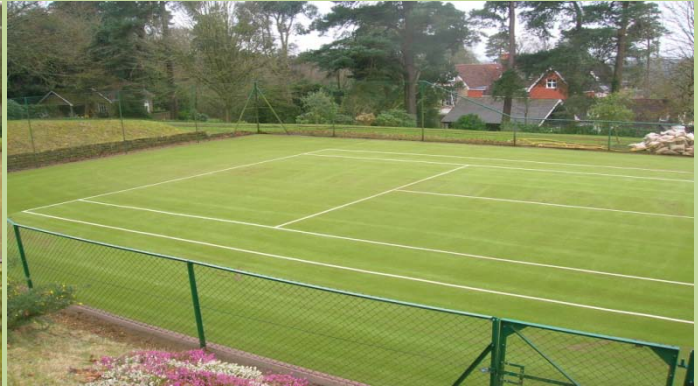
Tennis court after Rejuvenation with old infill extracted & new applied
