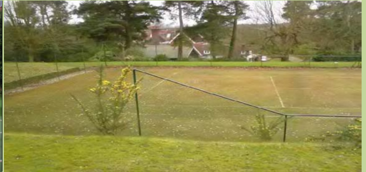
Moss can establish itself in an artificial grass court if not maintained
