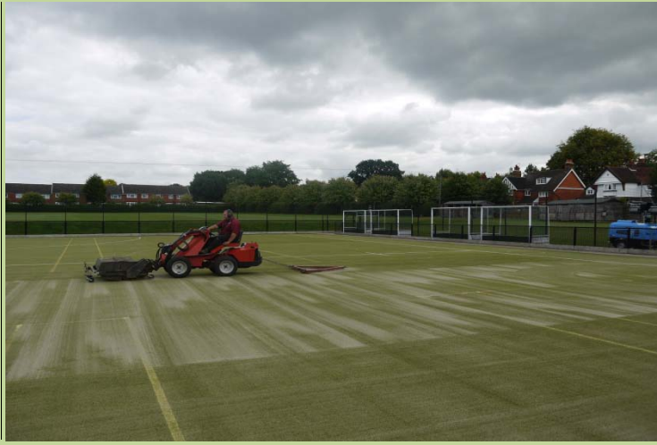
Astro turf pitch being infill decompacted
