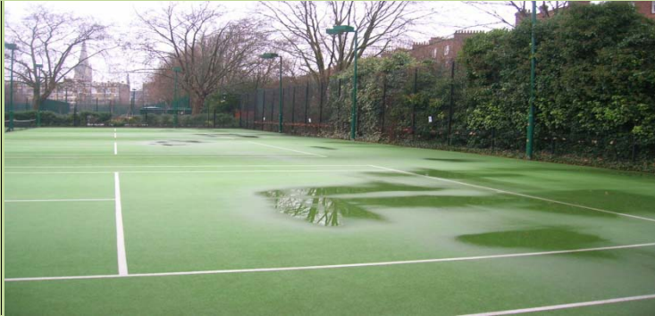
Infill compaction & contamination leads to flooding and poor drainage
