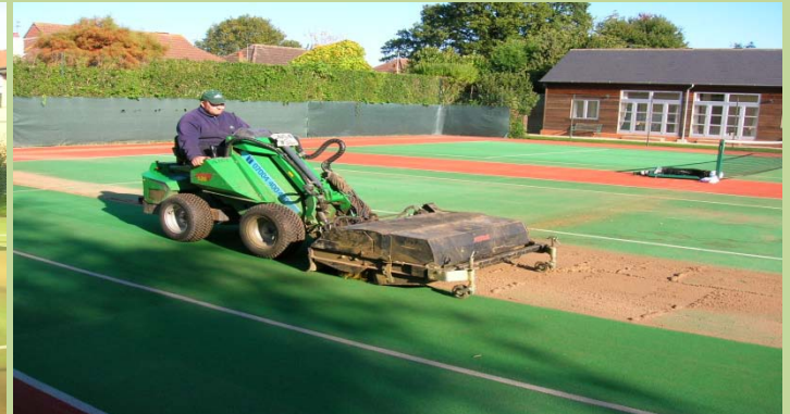
Decompaction of tennis court infill
