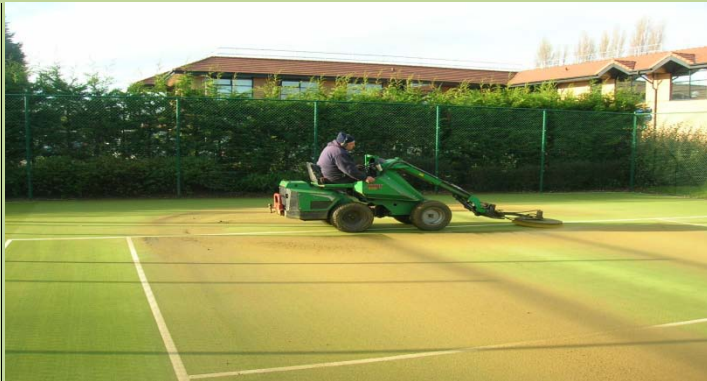
Decompaction of tennis court infill
