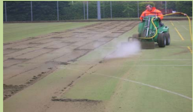
SSP Rejuvenation unit extracts the infill by a compressed air process
