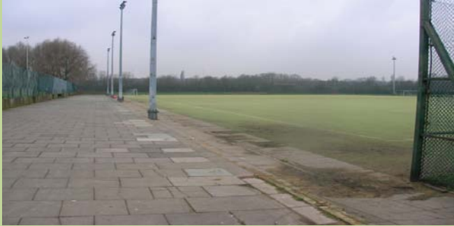
Astro turf pitch contaminated by moss & algae before Rejuvenation
