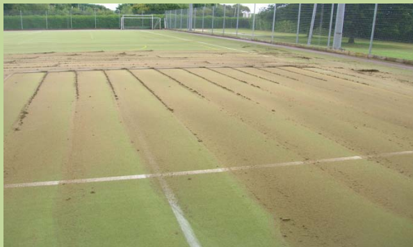
Step 2 – Collect the contaminated infill
