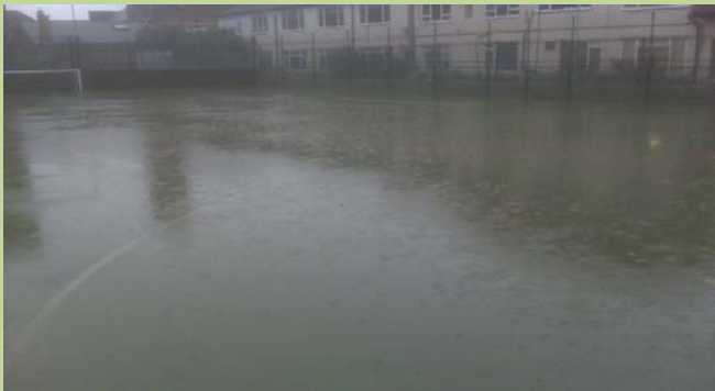
Infill compaction & contamination leads to flooding and poor drainage
