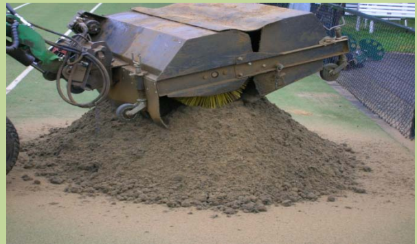
Step 4 – New infill is applied to the artificial grass
