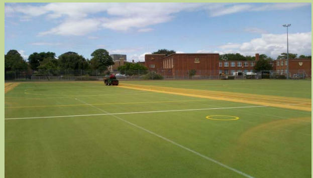
Step 4 – New infill is applied to the artificial grass
