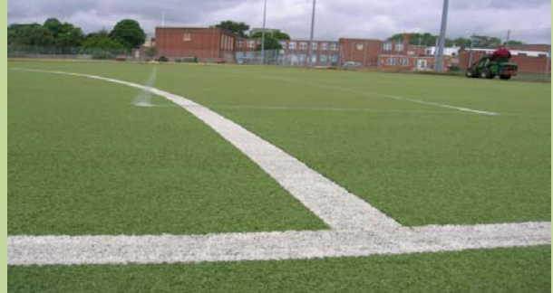
Astro turf pitch after Rejuvenation with old infill extracted
