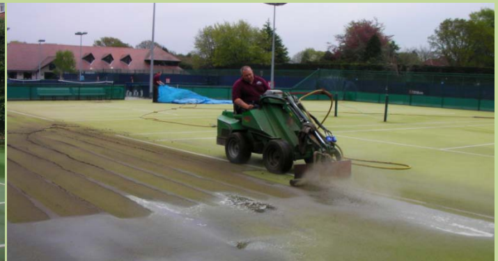
SSP Rejuvenation unit extracts the infill by a compressed air process
