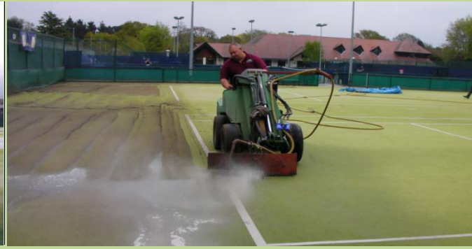
Rejuvenation unit using compressed air to extract contaminated infill
