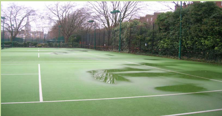
Infill compaction & contamination leads to flooding and poor drainage
