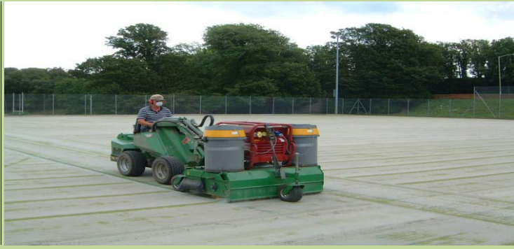
Astro turf pitch being cleaned and infill decompacted
